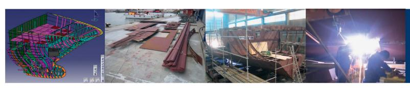
A year in the life of a 45m build: from initial CAD designs, 4,000 parts are cut ready for assembly to begin at the yard. Over the course of 12 months, the Viudes 45m starts to take shape. Far right: CFD work ensures an
