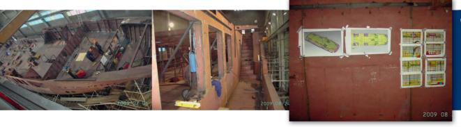
While work continues on the main hull and superstructure build, a full-size mock-up of the interior allows for refinements to be made, as well as giving the owner a chance to make modifications to the general arrangement
